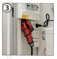
Connect the power cable and turn on all switches. If the trailer has a macerator pump, connect it and switch it on.
