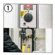
First, turn off the water heater and disconnect the water supply. (It must not be switched on without water)
