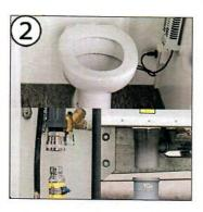
Empty all toilets by flushing them one last time. Then disconnect the sewage connection.
