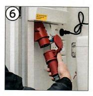
Finish by disconnecting the power cable. Remember to clean the trailer if you have rented it.
