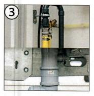
Connect the hose/sewage pipe. If the toilet has a macerator pump, remember to connect it and turn it on.
