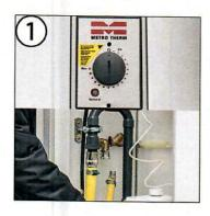
First, turn off the water heater and disconnect the water supply. (It must not be switched on without water)
