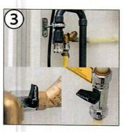
Connect the water hose and close all drain cock valves. Turn on the water and then the main tap.
